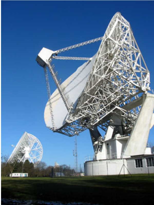
This is a photograph of two of the Jodrell Bank radio telescopes (the 76-metre Lovell Telescope in the background and the 25-metre Mark II telescope in the foreground) that were used to observe the recurrent nova RS Ophiuchi as part of the European VLBI Network observations, which have shed new insights into what happens when stars explode. (Image Credit: Tim O'Brien, Jodrell Bank Observatory)
