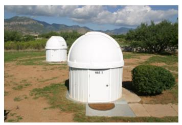
Hereford Arizona Observatory, used for observations of exoplanets (for XO and AXA projects), dwarf eclipsing binaries (for Vanderbilt University) and white dwarf monitoring for exoplanet transits. One dome houses a Celestron 11-inch (CPC-1100) telescope, and the other houses a Meade 14-inch (LX-200GPS). Both are controlled using buried cables. The domes are 8-foot-diameter ExploraDomes, and are motorized for azimuth movement only.
